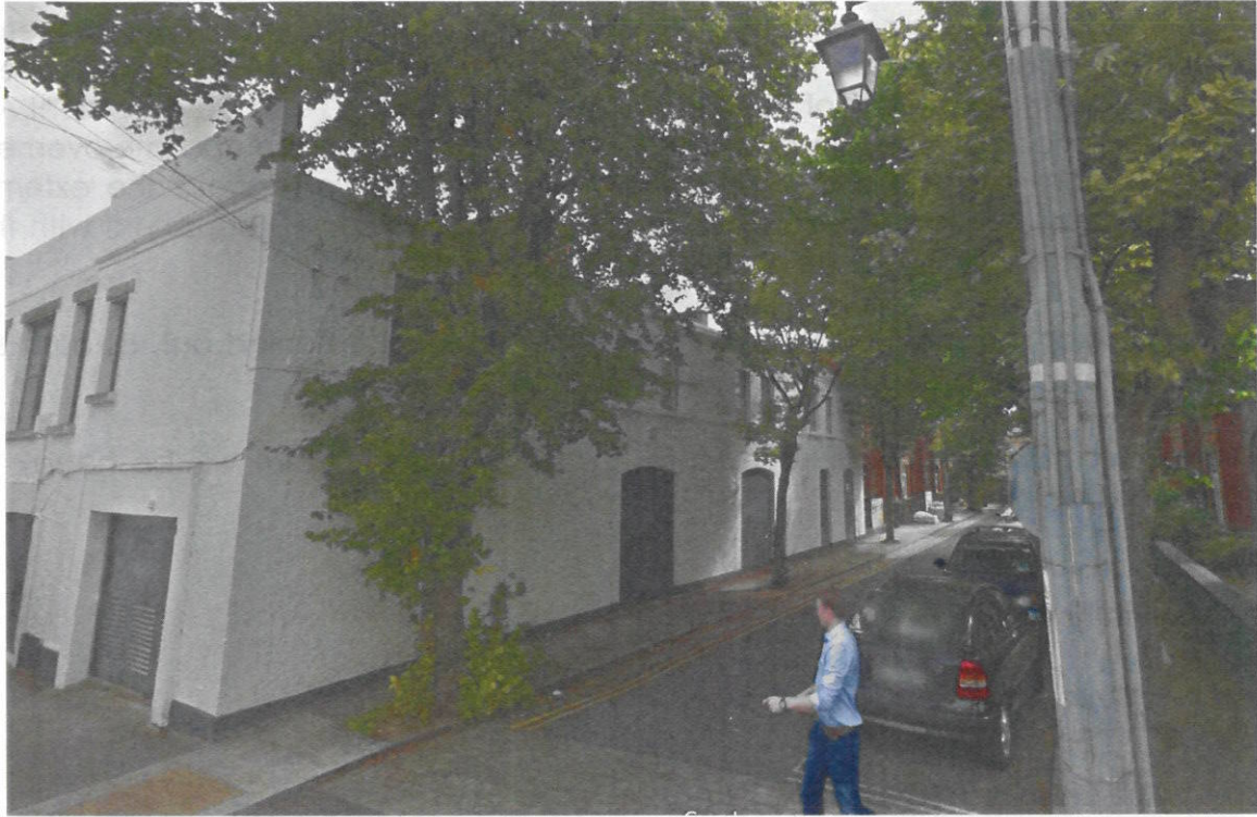
(Source: Google Street view Photograph August 2014)
